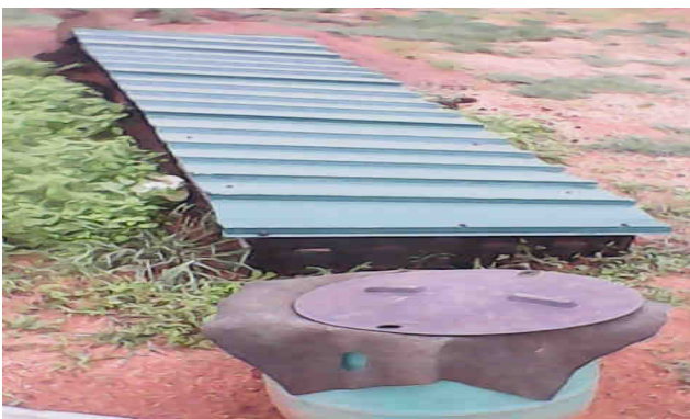
Fig 3 showing a tubular biogas digester in Lubombo
