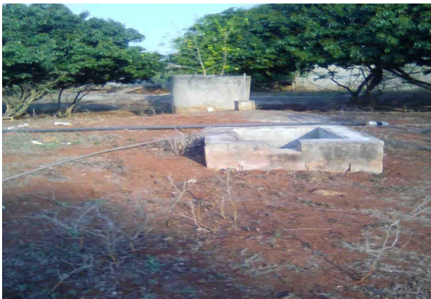
Fig 4 (a) showing a fixed dome biogas digester installed in 2012 at a piggy farm in Manzini
